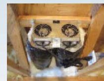
Between joist/truss mount
